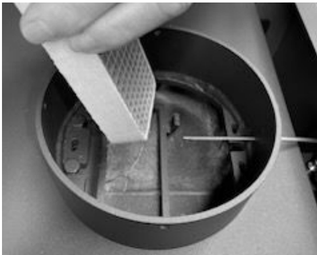
Figure 2: Insert combustor into flue.
